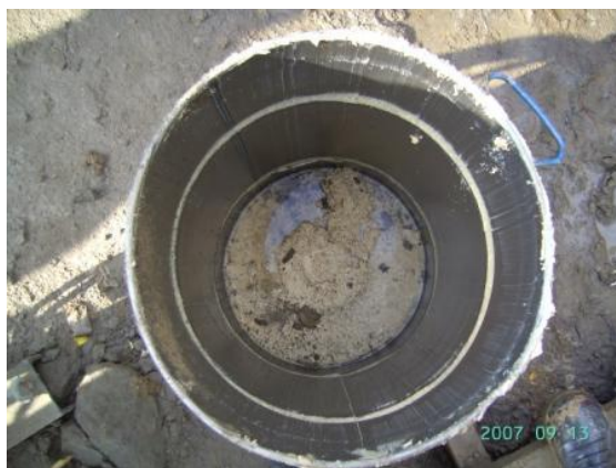
Empty drum after pumping
